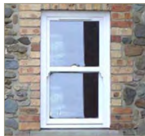
Window with Clear Glass & Trickle Vent
